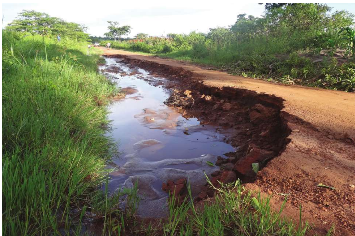
Plate 2: Eroded section of Gogonyo road, Pallisa District
